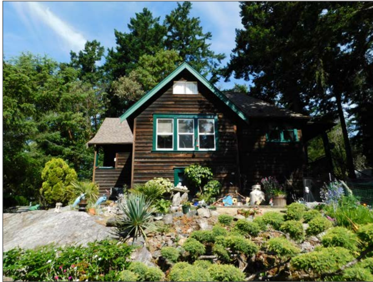
Photo 1 – View of the south elevation of Site Building A.
