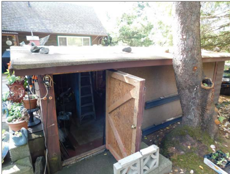
Photo 2 – West elevation of Site Building B.
